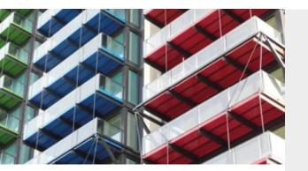
Designed by ROGER STIRK HARBOUR AND PARTNERS the Merano residencies at the Albert Embankment London consists of 40 luxury apartments overlooking the Thames. MACALLOY BALCONY HANGERS were used in various inclinations to support the balcony deck anchored into the structure using a "gallows" concept giving an Aesthetic feel and design. This solution maximises the floor area and gives a large viewing platform across the Thames.
